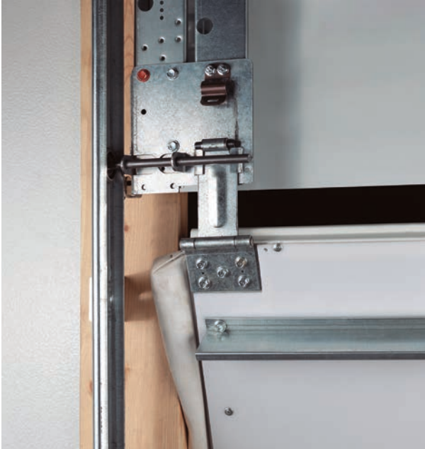
Inside View of Single Bottom Section
